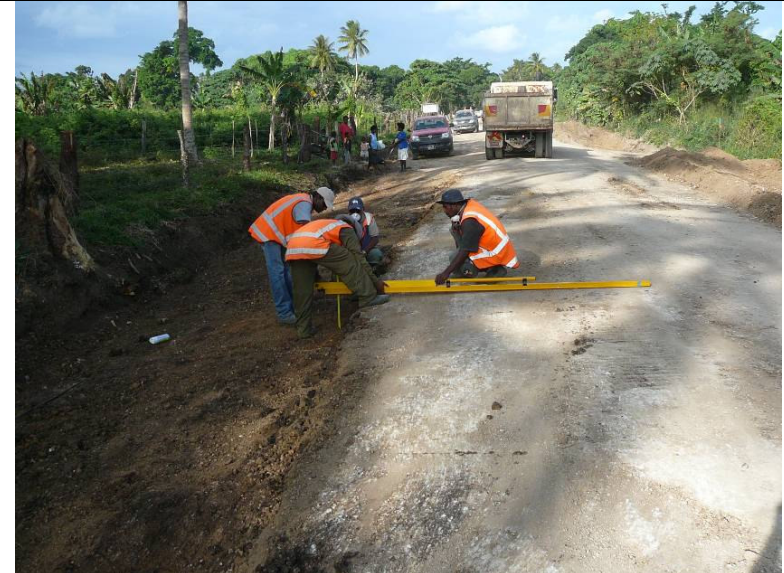
Checking depth of excavation, Site Engineer Bhan Prakash (left) with ESU Supervisor James Hakwa (rear), with Stewardson Bihu & Isaiah Tonlong..
