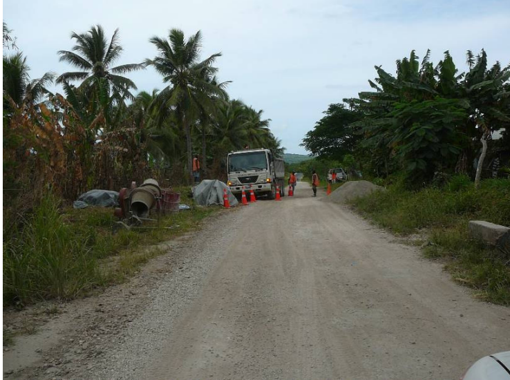
Starting work in the Tanoliu section. The Drainage crew getting ready to install a culvert near Ulei.
