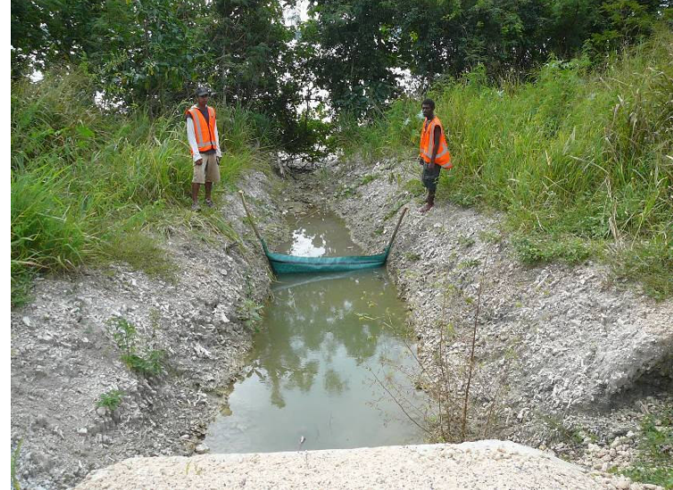
Environmental protection, Gregory Popovi (left) and Craig Kalkauo checking a partially completed silt fence near Port Havannah.
