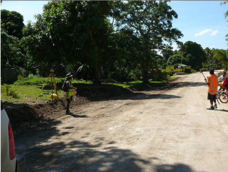
Emua on Saturday. Survey team checking levels after vegetation has been cleared and the road widened ready for the final basecourse layer.
