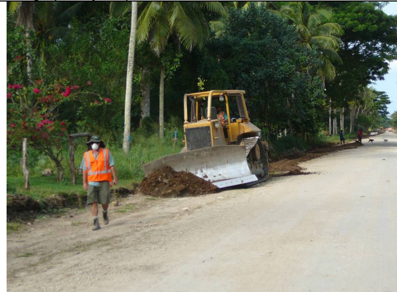
Follow me – Project Engineer Marcin Golucowski with the D6 bulldozer operated by Max Kai forming a side drain near Safaki - on a dry dusty day.
