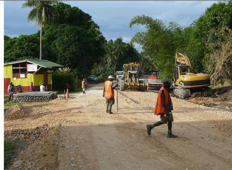
Emua on Wednesday. Pavement crew placing the final basecourse layer past the Ground Breaking Commemorative Plaque (stone plinth on left).
